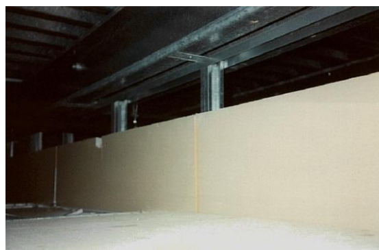
Vertical compartmentation not extending up to floor slab above (incorrect)
