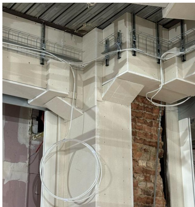
Board fire protection to steel
