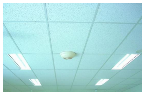
Typical suspended ceiling system
