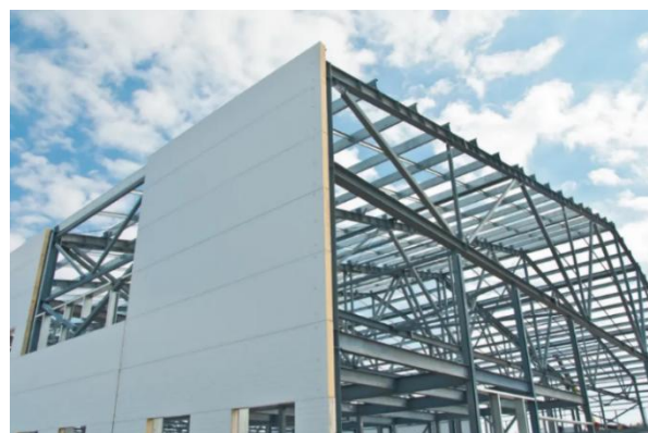
Tall buildings in warehousing/food factories constructed from sandwich panels
