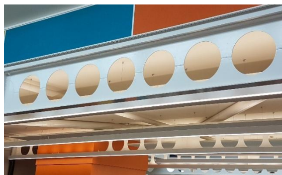
Intumescent/reactive coating on cellular beams
