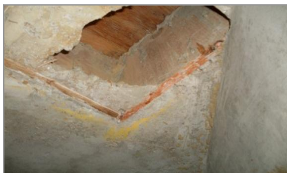
Compartment floor with a hole passing through to the laminate floor in the flat above (incorrect)
