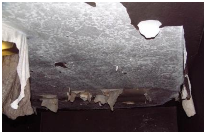
Poor adhesion can lead to rapid flame spread
