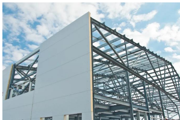
Sandwich panel construction building
