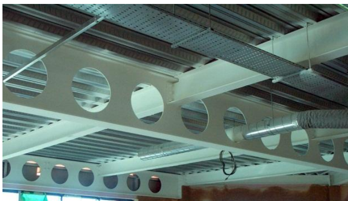
Intumescent (reactive) coating on cellular beams
