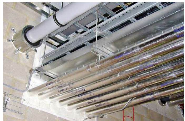
Figure 20 Multiple services within a single aperture. Lower services limit the access to the upper penetration seals
